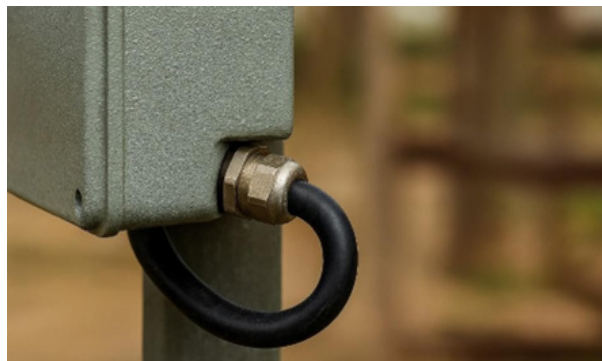
Figure 2: Proper cable gland installation with drip loop and double compression sealing
